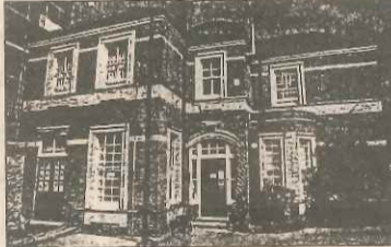
Contact point: the headquarters of the ICA in west London
